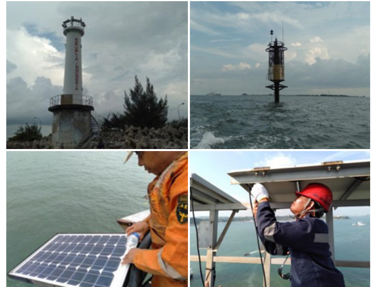
Solar Cell installation for Navigational Aids (SBNP) in the Strait of Malacca and Singapore
