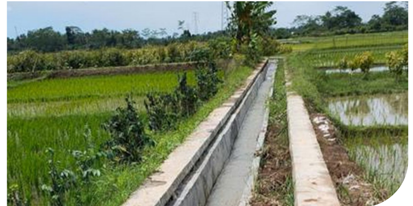
Note: Tertiary irrigation canal in Seberang Kapuas Village, the District of Sekadau (the Province of West Kalimantan). Source: Kompas
